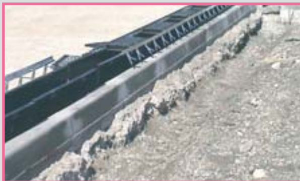
(Fig. 1) • MufleDrain installation underlying layer
